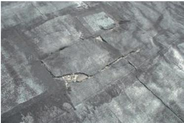
The existing bitumen roof had to be renovated completely because it no longer complied with the required wind load. The presence of holes and tears had made the roof covering very rough. To ensure that the Hertalan EPDM roof covering could be laid properly and flat, the choice was made to affix an additional insulating layer on the existing bitumen roof covering.
