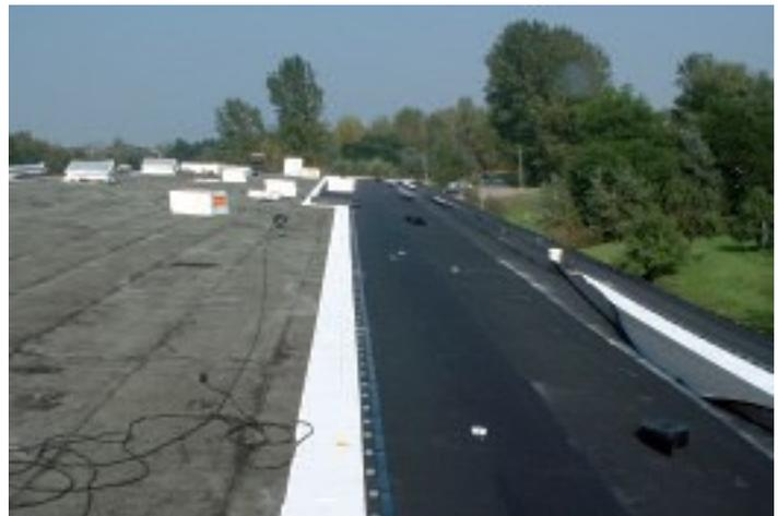
Hertalan easy weld MF is a mechanically fixed system of roofing rolls, where the seams are sealed with hot air. Hertalan developed a unique EPDM roofing strip with a EW welding seam for this system, whereby the EW seam is UV resistant.
